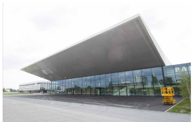
ETFE cladding exterior canopy Bordeaux
