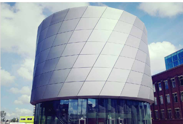
Facade cladding This Is Holland pavilion
