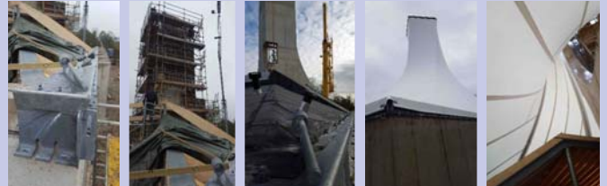
Pictures of construction process © Buitink Technology
