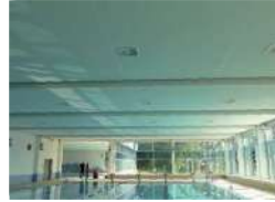
Tensioned ceiling - Aqua centre (CH)
