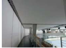
Ceiling and walls - Vaujany ice rink (FR)
