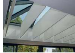
Ceiling and baffles - Restaurant (FR)
